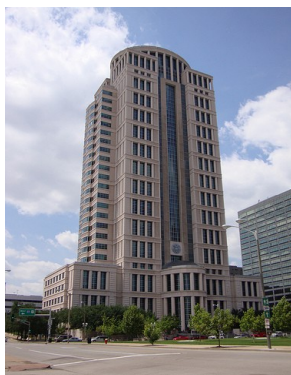
Thomas Eagleton Federal Courthouse. It is the largest courthouse in the country.
